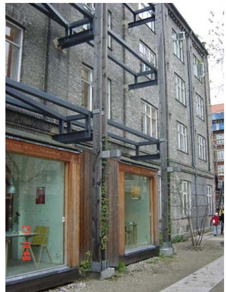
Children's library in a former factory from the centre of Copenhagen - façade
